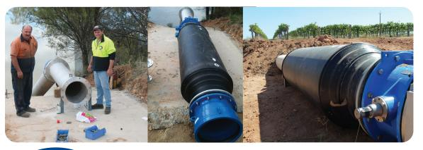
Riverland grape grower Dino Sigismondi, right, starts to install a DELTA SU450 SL501 onto a 450mm pipeline on the Murray River 30 kilometres down river from Loxton, SA. The pipeline irrigates a 121-hectare vineyard.
